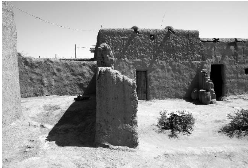
Fig. 9: Multiple episodes of building and modification are visible in the mudbrick fabric of the Basheere family's compound (photo: C. Kleinitz)
